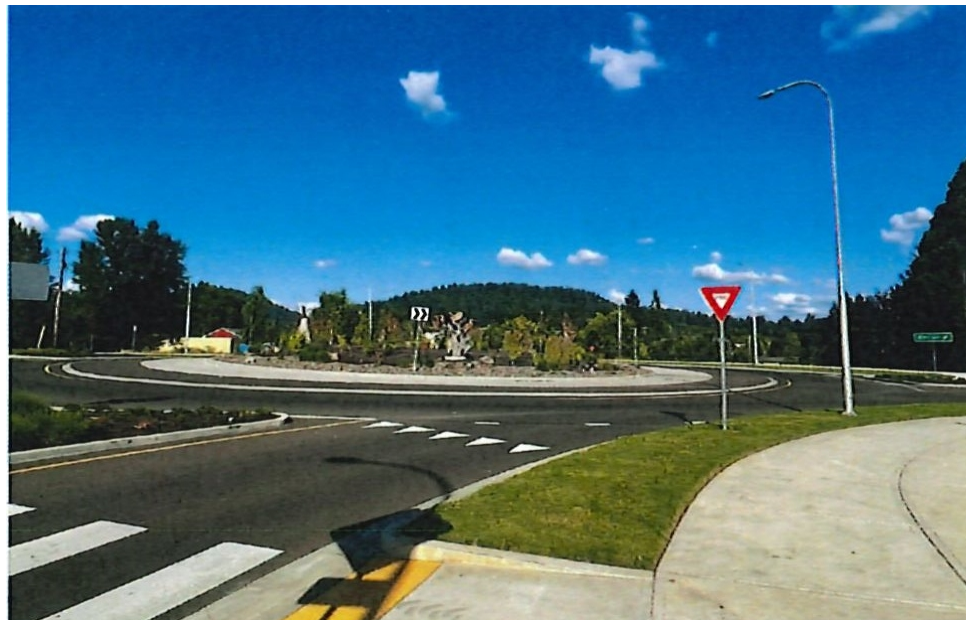
Typical Visual of a Roundabout Similar to the finished product at Badger and South Canal.
