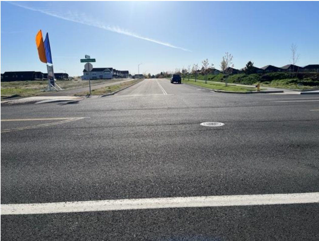
Figure 16. View from NW Spruce Avenue facing east toward the Dry Canyon PUD.
