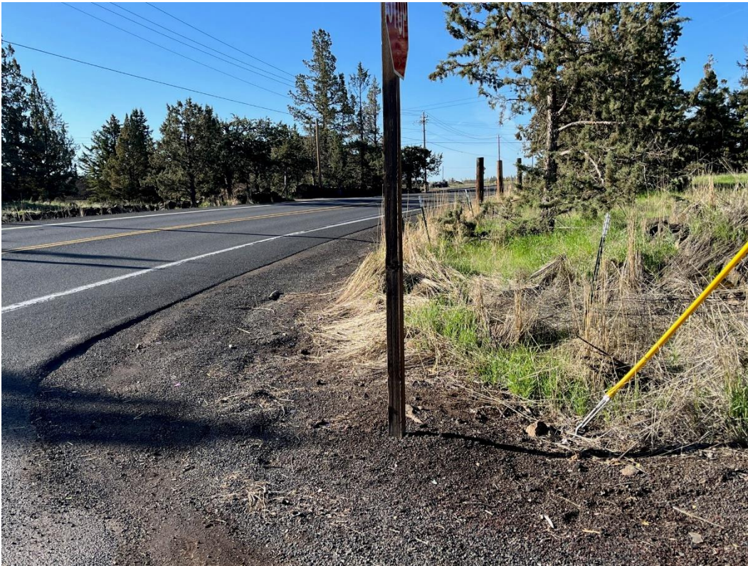
Figure 10. NW Northwest Way/NW Upas Avenue facing south.
