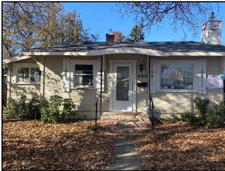
525 SW 10 th Street viewed from 10 th Street (2023)
