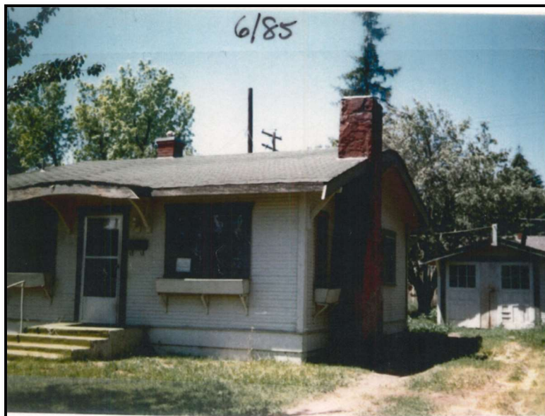
525 SW 10 th Street viewed from 10 th Street (1985)
