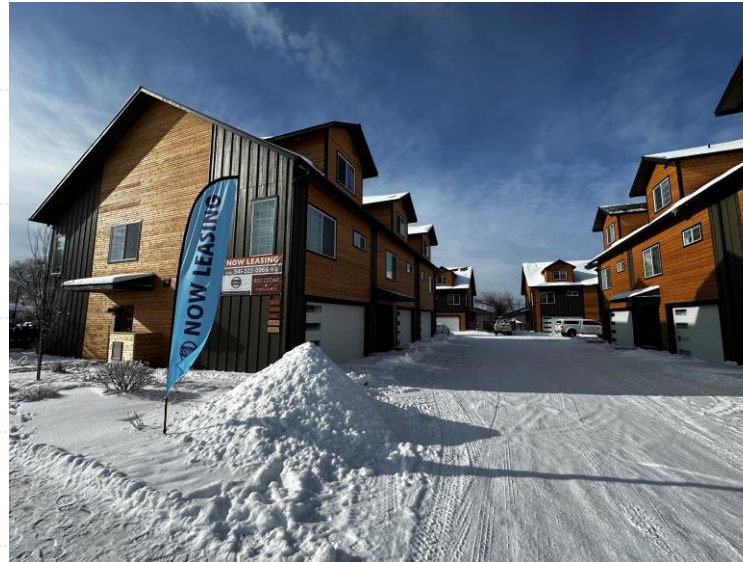
4 th St. Project
