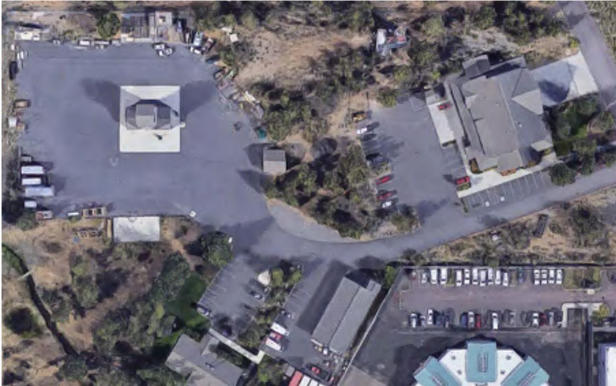
FIGURE 1 - OVERVIEW OF BEND FIRE AND RESCUE TRAINING FACILITY
