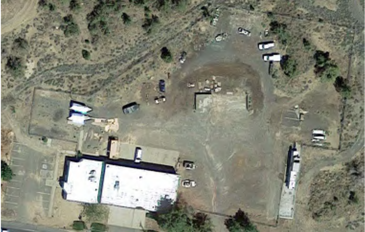
FIGURE 3 - OVERVIEW OF REDMOND FIRE AND RESCUE TRAINING CENTER
