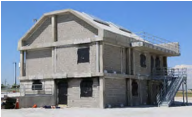
FIGURE 19 - MULTI STORY BURN BUILDING, AURORA, CO
