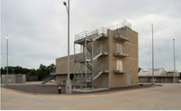
FIGURE 16 - DRILL TOWER, AURORA CO
