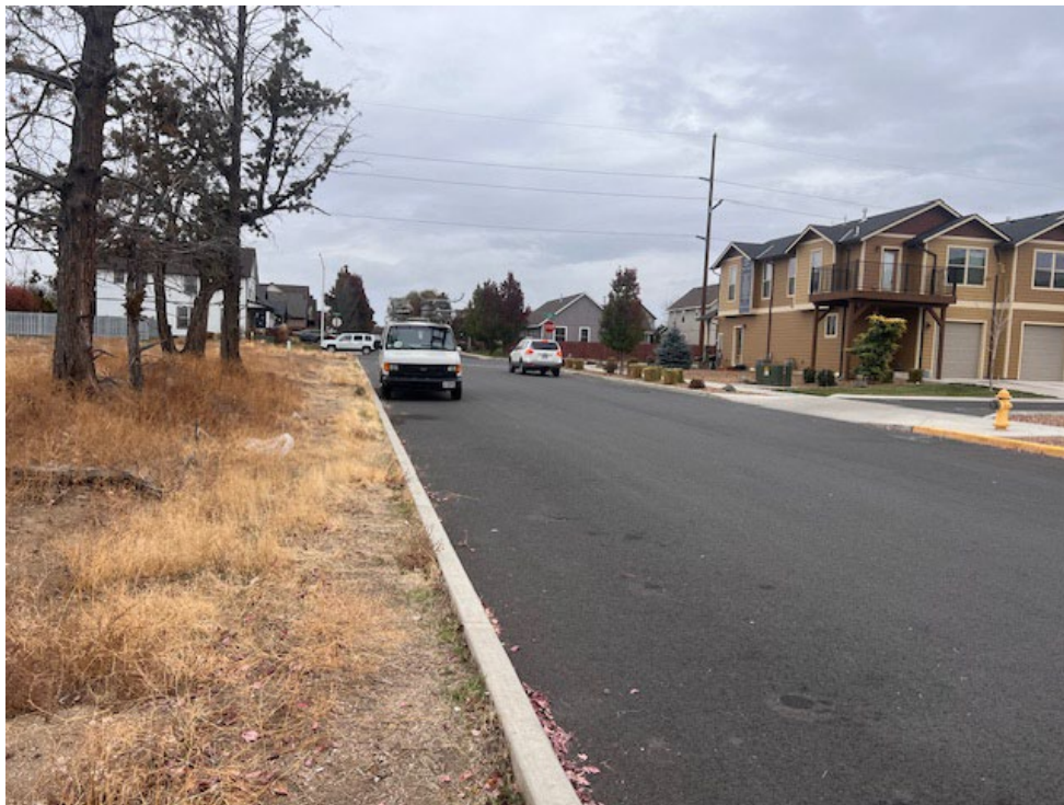
Looking east from the east access. The available line of sight to 35 th Street, which is sufficient
