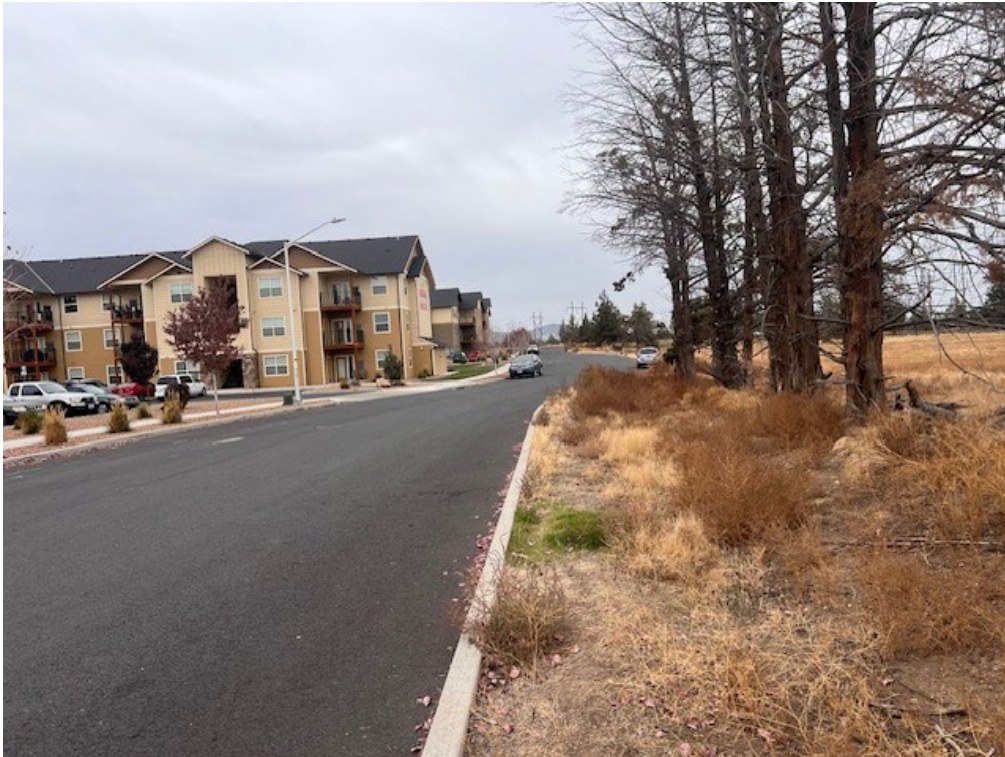
Looking west from the east access. The available line of sight to 37 th Street, which is beyond 300 feet.
