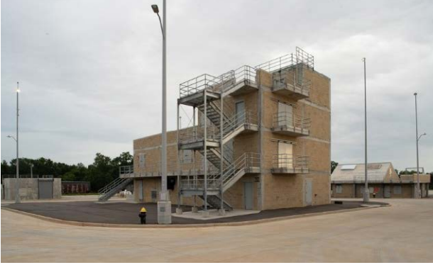
FIGURE 16 - DRILL TOWER, AURORA CO
