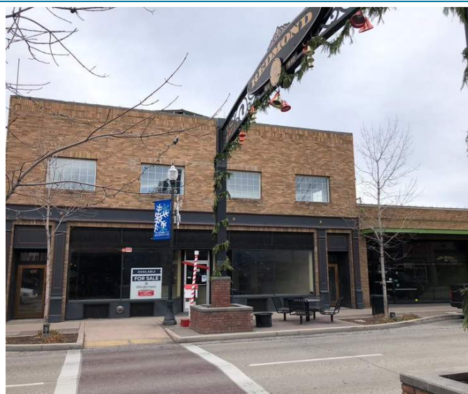
Existing Building Front
