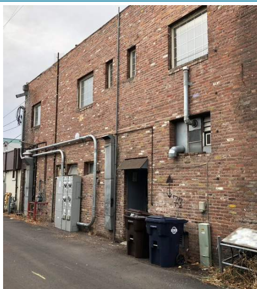
Existing Building Rear View
