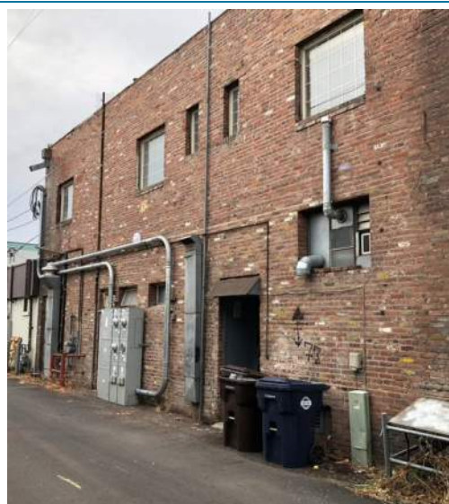
Existing Building Rear View
