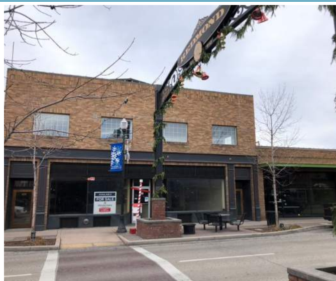
Existing Building Front
