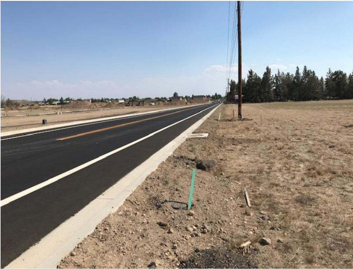
Figure 9. NW 10 th Street facing south.
