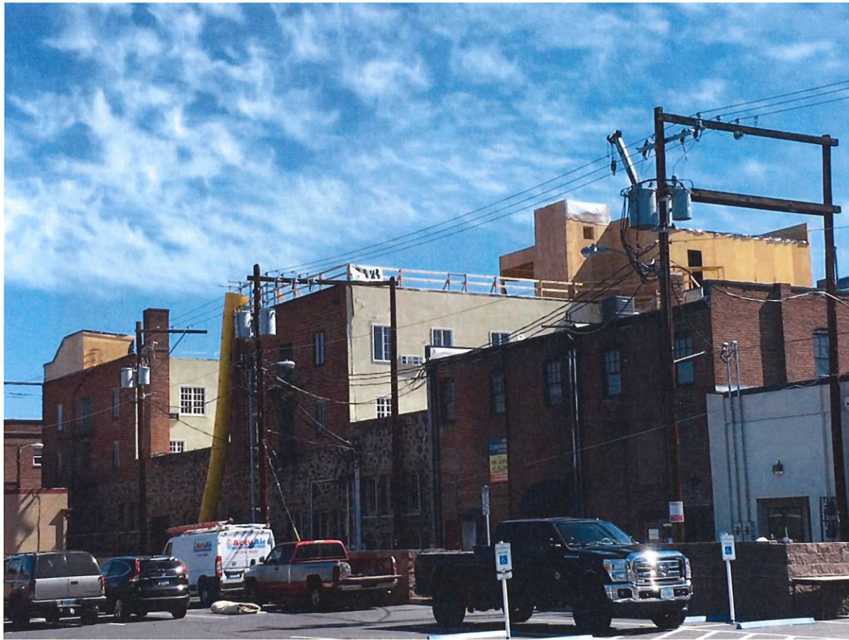
Taken from 7 th and Forest. The addition is visible, but view is marred by existing power lines and not a primary viewpoint.
