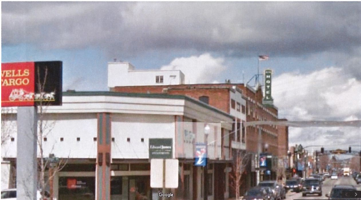
Photo of previous elevator structure on top of the hotel that shows there was building mass originally located on top of the structure and which is being replaced by a new structure.
