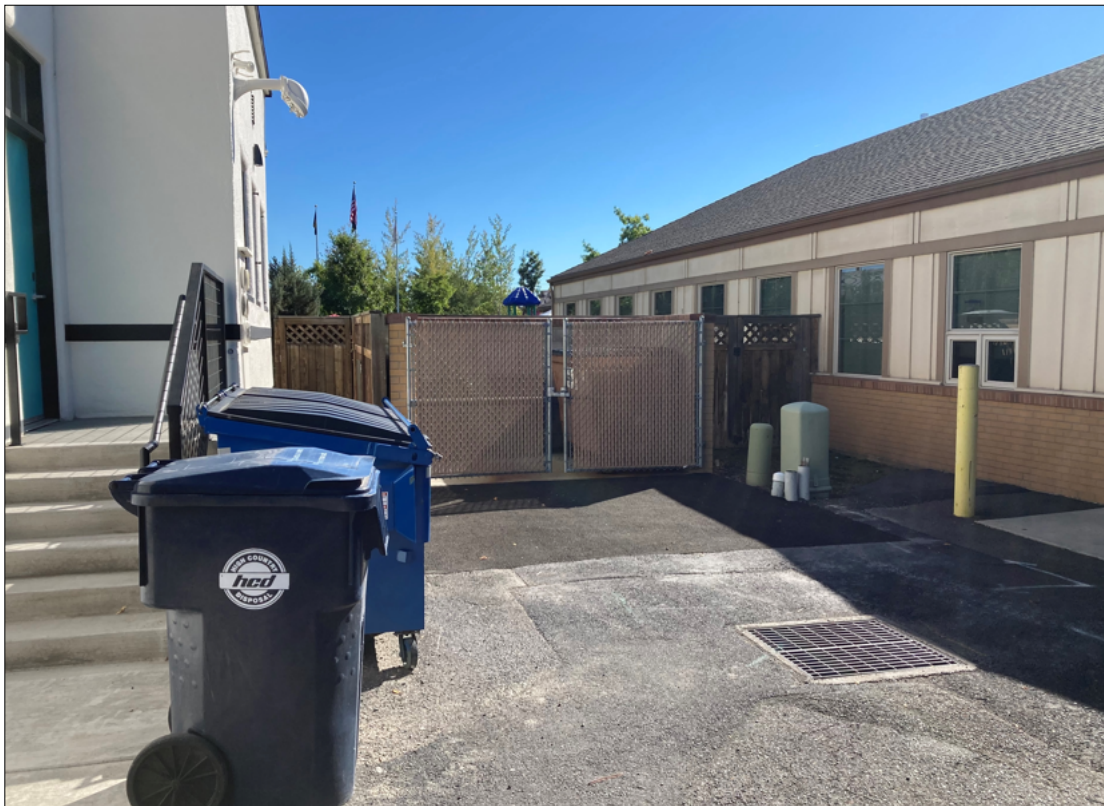
Picture – Existing Trash Enclosure / Alleyway
