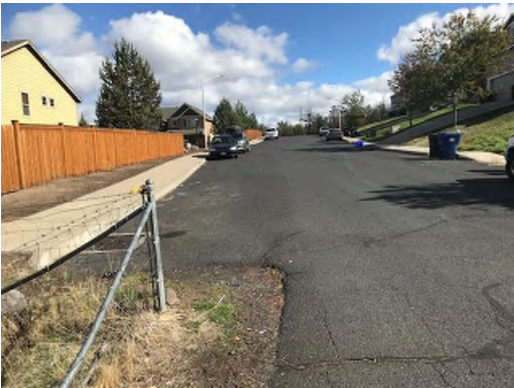
Figure 8. SW 42 nd Street connection to SW Reindeer Avenue facing east.
