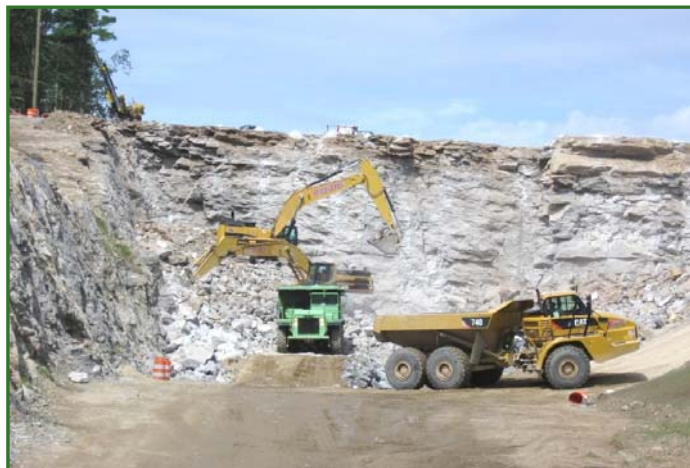
ROCK & LEDGE REMOVAL OPERATIONS
